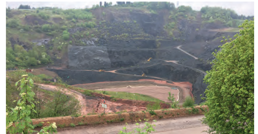
View from within the site looking north over infilled quarry area
