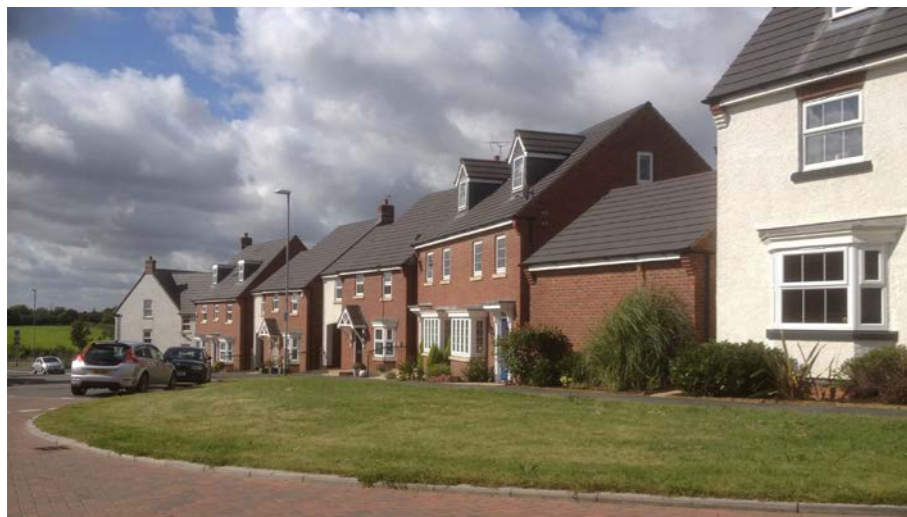
Positive housing frontage
