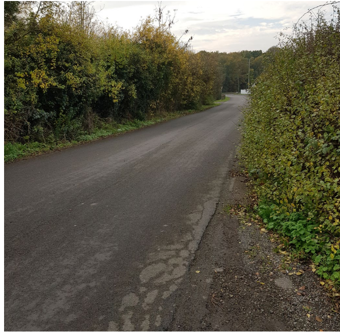
Brick Kiln Lane looking north
