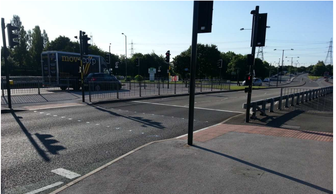
Figure 8. A34 south, junction with Chapel Lane (08:19 22/07/14)
